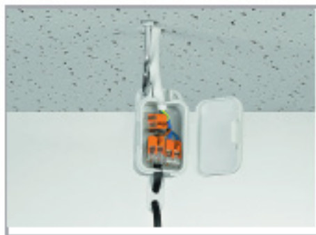
Pendant light connection in suspended ceiling
