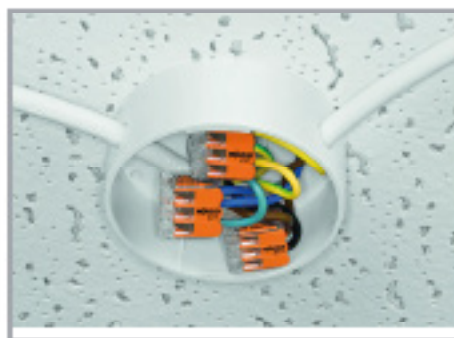
Lighting distribution in ceiling canopy
