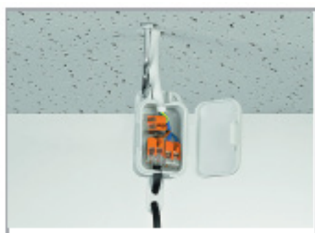
Pendant light connection in suspended ceiling
