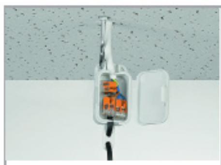
Pendant light connection in suspended ceilings
